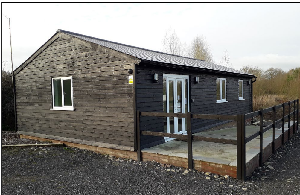
Figure 6 – Existing amenity block
