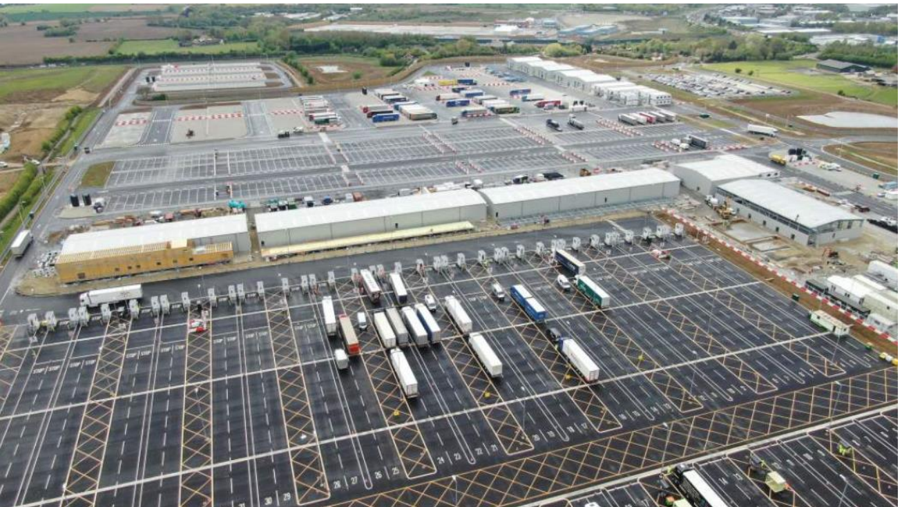
View from the North. Office buildings under construction to left of picture – to rear of inspection sheds.
