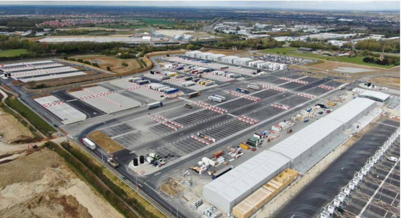
Southern section of site showing HGVs at HMRC offices
