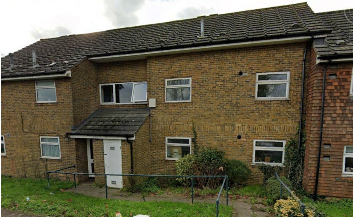
Figure 3 - Existing north east entrance on Newton Road
