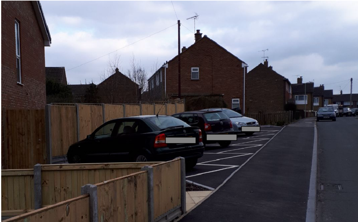
Figure 4 Parking as built.
